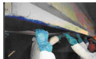
(e) Manual Lay-up of CFRP Sheet
