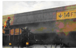
(b) Surface Sandblasting
