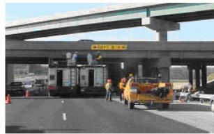
(a) Overall View
