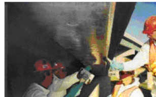
(c) Application of Putty
