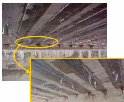
(b) Bolted CFRP Plates
